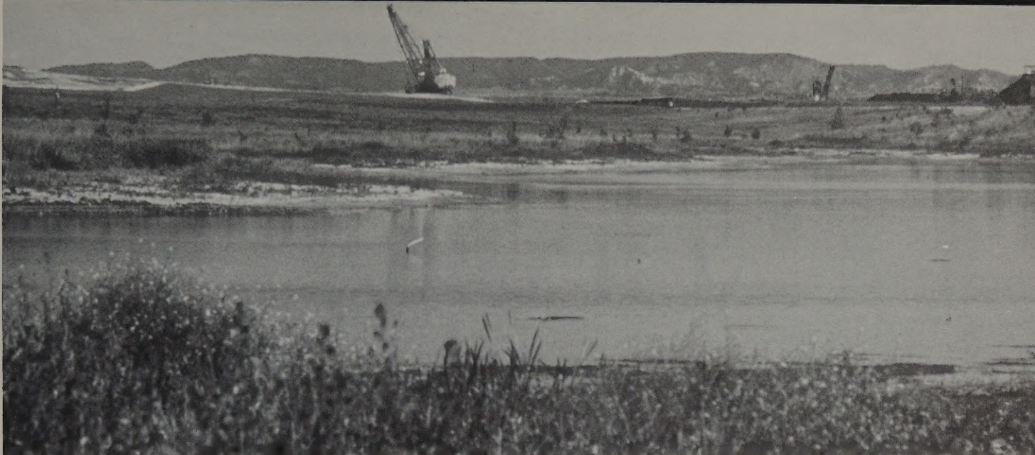
All water used in mining must be contained on the site and is usually collected in a sediment pond such as this. Aquatic plants and native trees including green ash, boxelder, chokecherry, and cottonwood enhance the shoreline. Ten thousand largemouth bass were used to stock the pond, which also provides water for wildlife and livestock. Removal of federal coal from this site and cooperative reclamation actions created this public recreation area.
